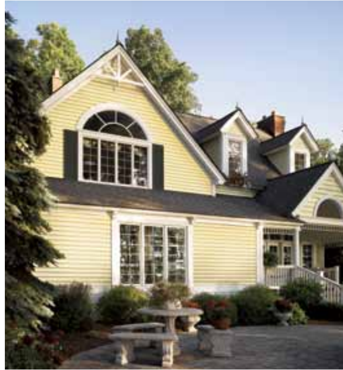
Siding: Monogram Double 4" Clapboard and Cedar Impressions Double 7" Straight Edge Perfection Shingles in autumn yellow Trim: Vinyl Carpentry® & Restoration Millwork®
