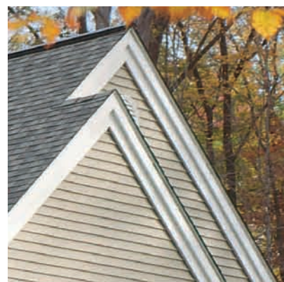
5" Trimworks lineals used as "rake" boards.
